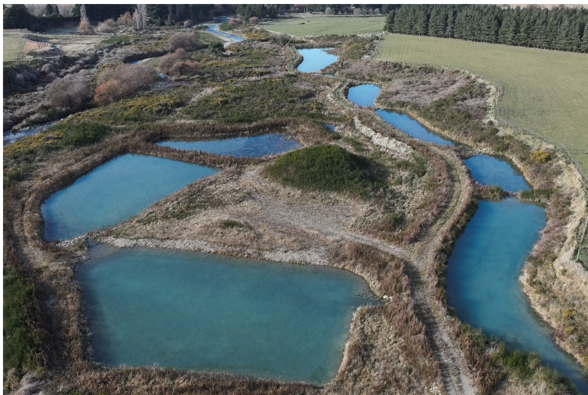
Figure 2-5: NRR1 2018 (right) & 2021 (left) recharge basins (Source: HHWET)
