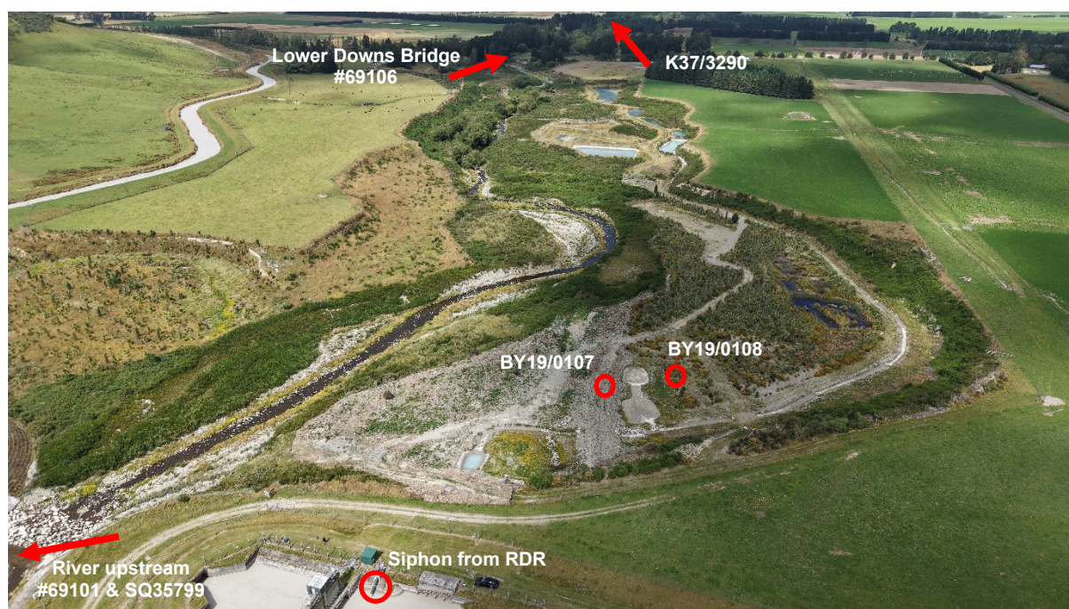
Figure 2-8: NRR1 monitoring points (Source: HHWET)
