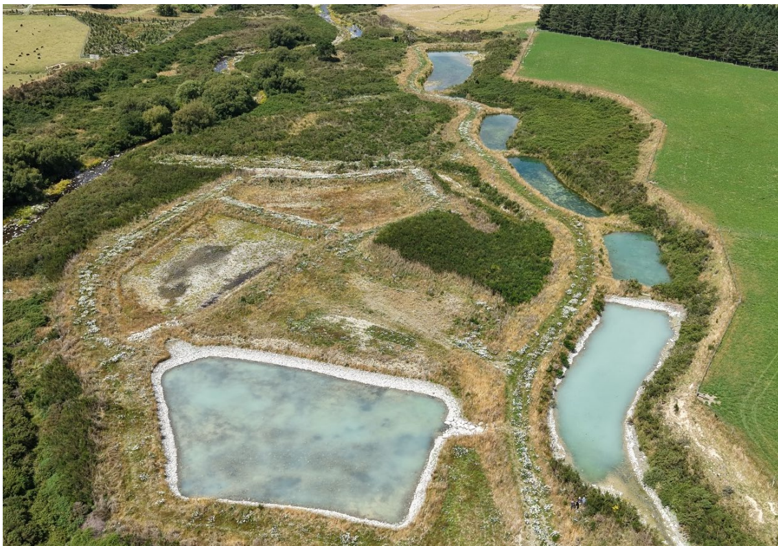
Figure 2-5: NRR1 2018 (right) & 2021 (left) recharge basins in January 2026, with colour changes showing glacial sediment drop out through the system and 2021 basin system well below capacity (Source: HHWET)
