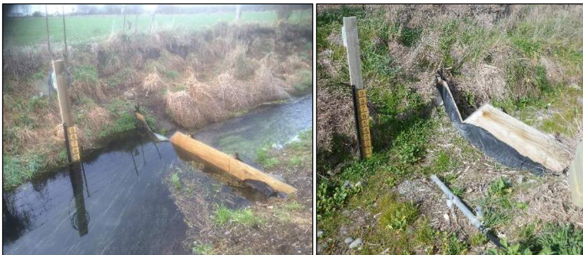
Figure E15: Parakanoi Drain MAR programme weir – comparison winter 2014 (flowing) vs winter 2016 (dry).
