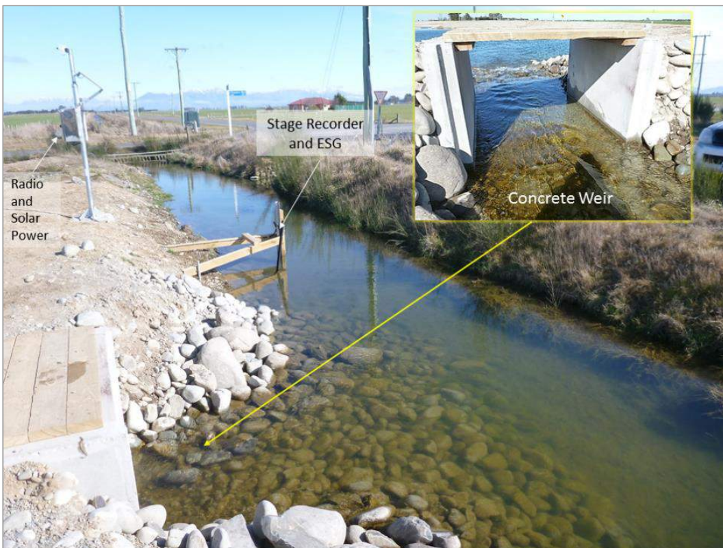
Figure E6: Flume 2 with ESG and logger structure.
