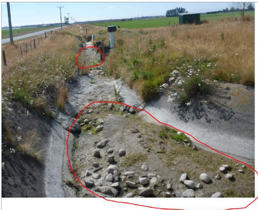
Figure L4: MAR race upstream from Flume 1 showing sediment deposited (red circles) during Year 1.
