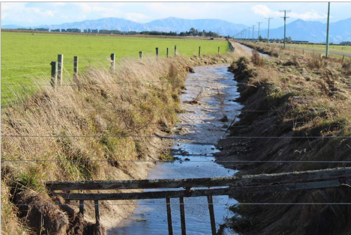
Figure L2: Open race delivering water source water to MAR Pilot Trial site (Race bypass and MAR site start up 1 , June 2016).
