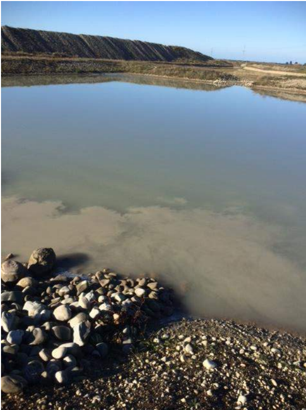
Figure I4: Sediment plume from inflow spillway to forebasin.
