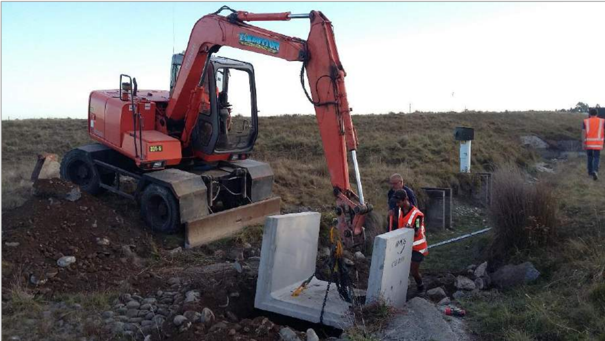
Figure L3: Flume 1 being installed downstream from the Valetta Pond #3 outlet (April 2016).
