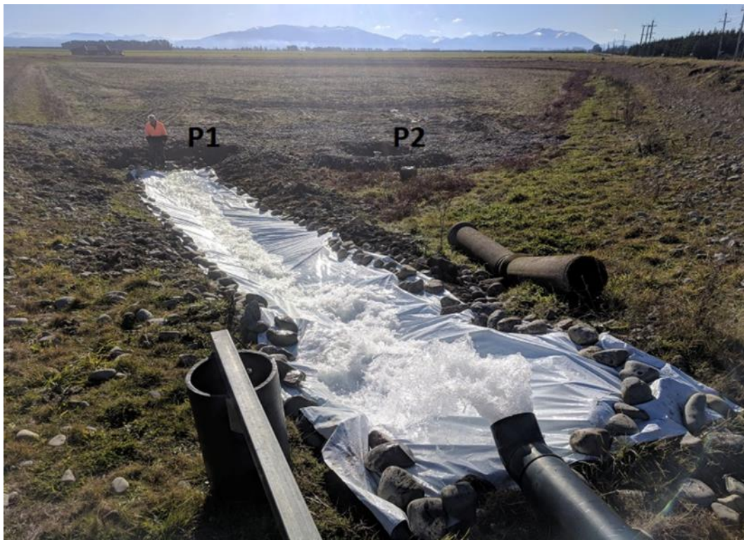
Figure F10: MAR07 site overview.
