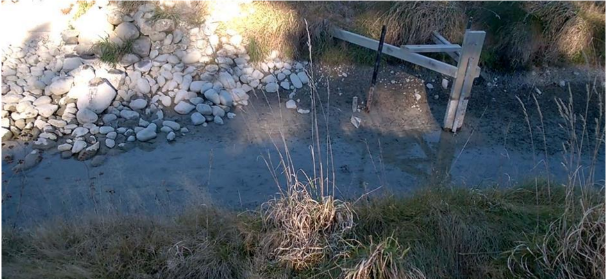
Figure D3: Photograph of delivery race floor (B. Painter, 18 July 2018).
