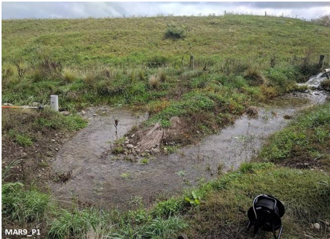
Figure F21: MAR09 site overview.
