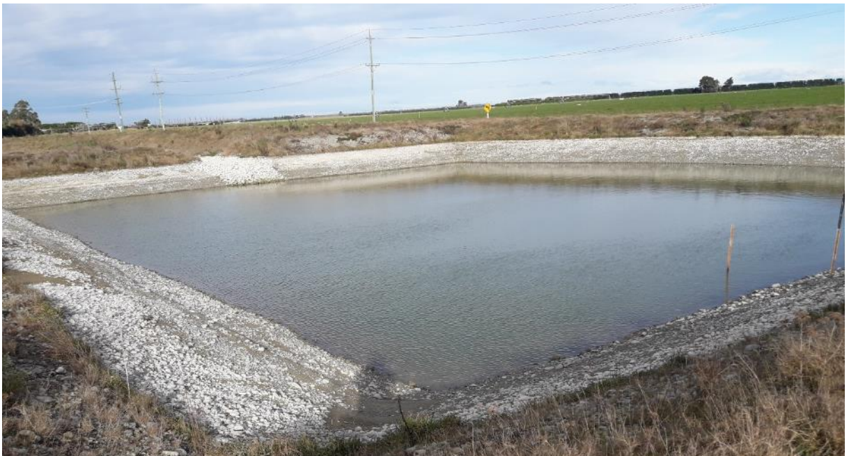
Figure D4: Settling basin (forebay) five days after flow to the Lagmhor Trial site ceased (9 July 2018).
