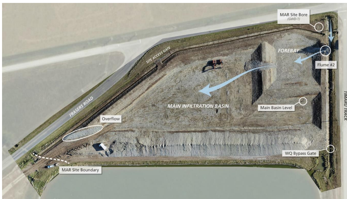
Figure 3: Lagmhor Trial site overview (from Golder 2017).
